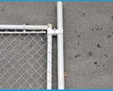
Step 8- Attach the second post to the other side of the panel with two more clamps.
